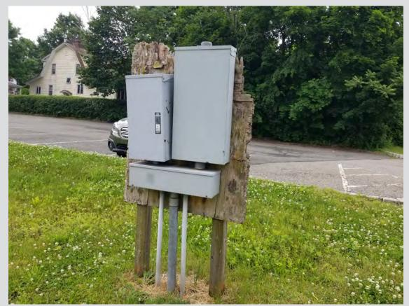
6. Electrical units on rotting plywood
